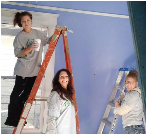
MBAG volunteers at work on final painting projects at JSCF.
