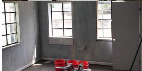
Before and near completion of renovation at Wilderness Works City Camp.
